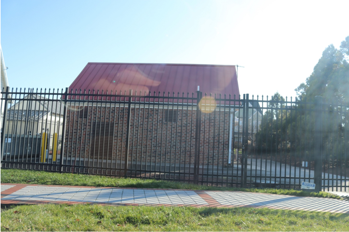
White's Heritage (Stoopley-Gibson), Gibson's Grant subdivision, pumping station, northwest elevation, looking southeast
