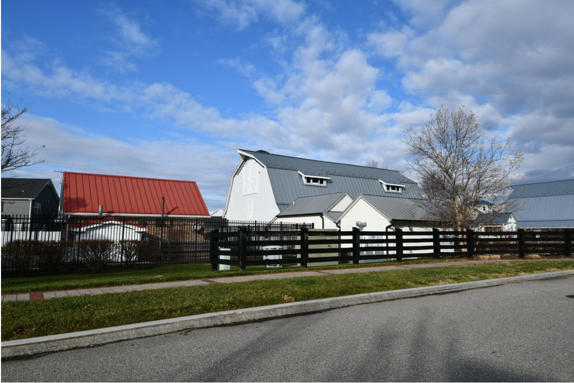
White's Heritage (Stoopley-Gibson), tenant farm complex, looking north
