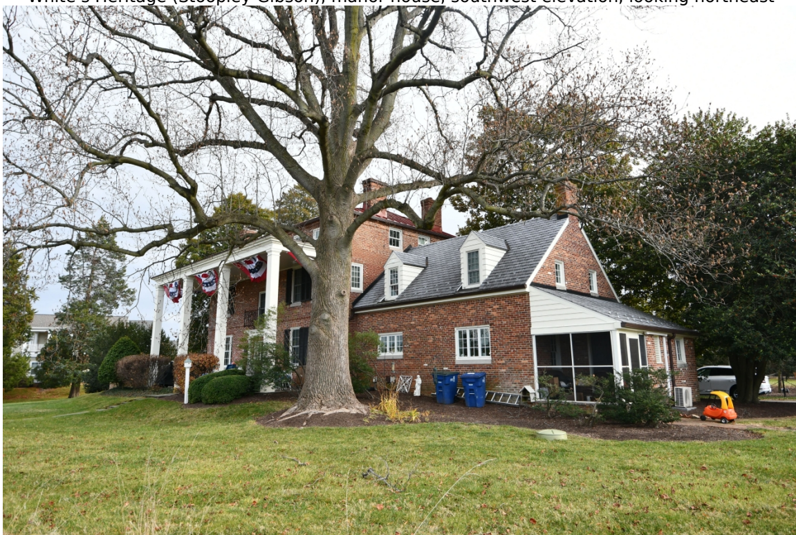
White's Heritage (Stoopley-Gibson), manor house, northwest and southwest elevations, looking southeast
