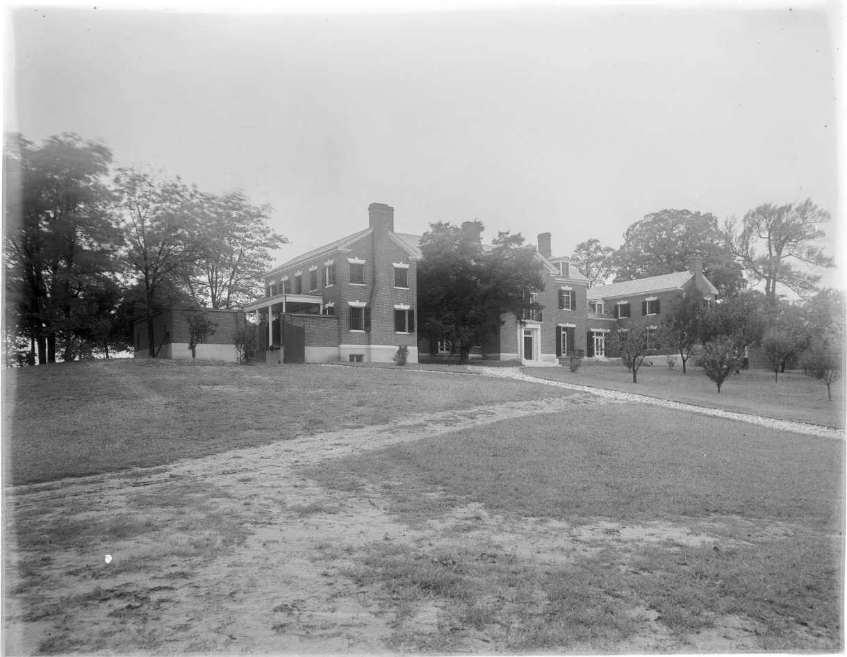
Historic Image 8: Photograph of Holly Beach Farm, looking west at the house and grounds. Photo Source: Sears, Thomas Warren. MD086043: [Holly Beach Farm]: the house and grounds. 1914. Thomas Warren Sears photograph collection, 1900-1966. Smithsonian Online Virtual Archives. https://sova.si.edu/record/aag.srs/ref4413?q=* .
