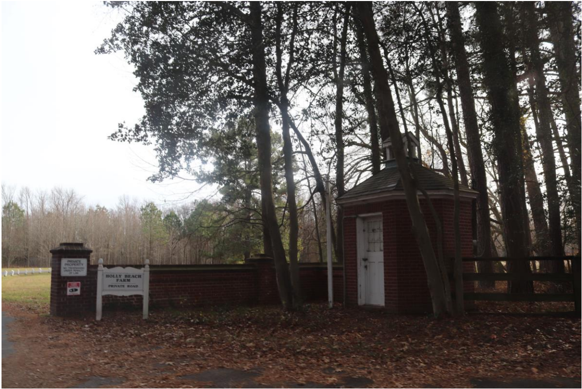
Photo 1 of 35: 1917 Holly Beach Farm Road, Gate House, Northwest Elevation, looking southeast
