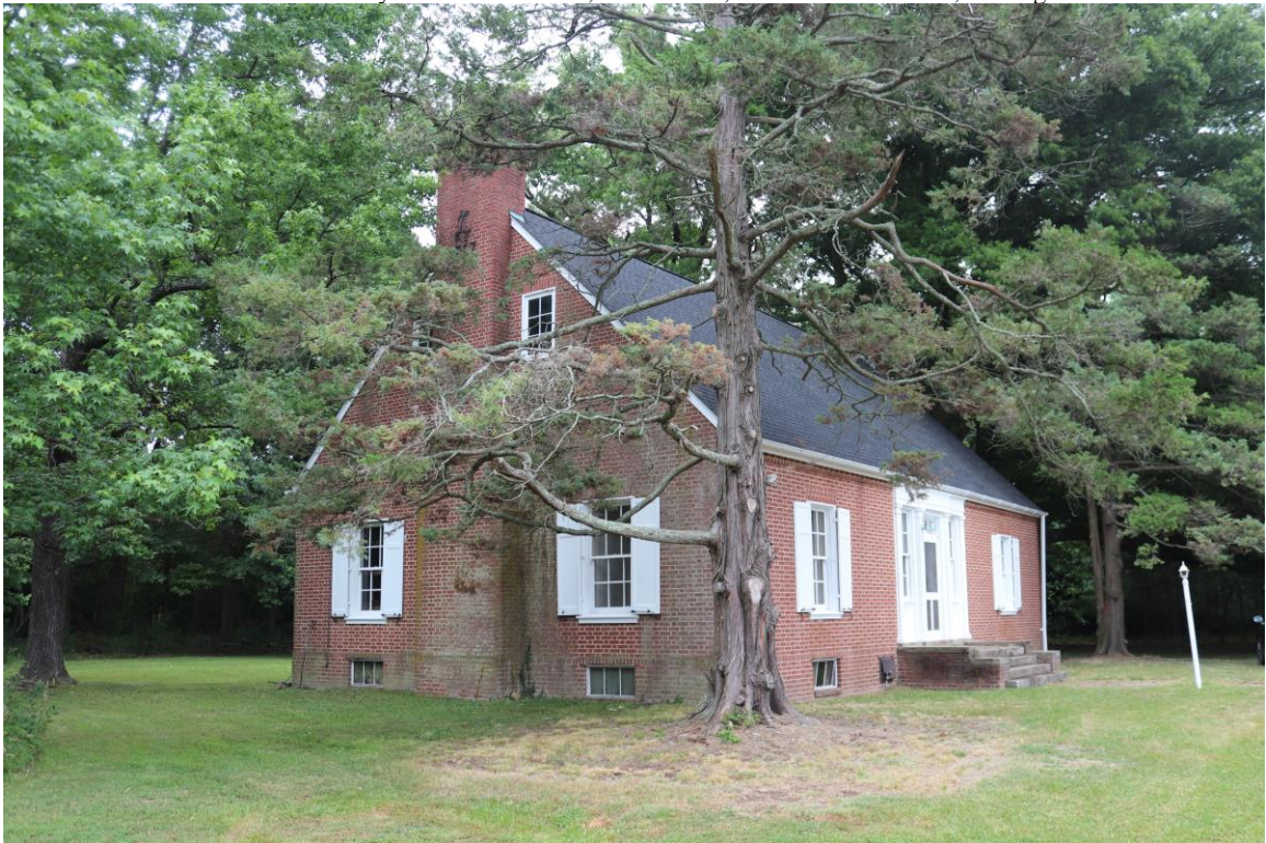
Photo 2 of 35: 1917 Holly Beach Farm Road, Farm Office, Northwest Elevation and Southwest Façade, looking northeast
