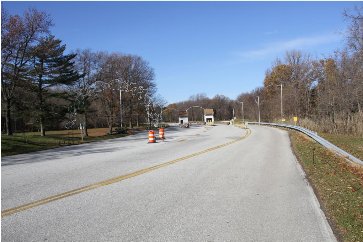
Photo 15 of 39: Park Gates, looking northwest
