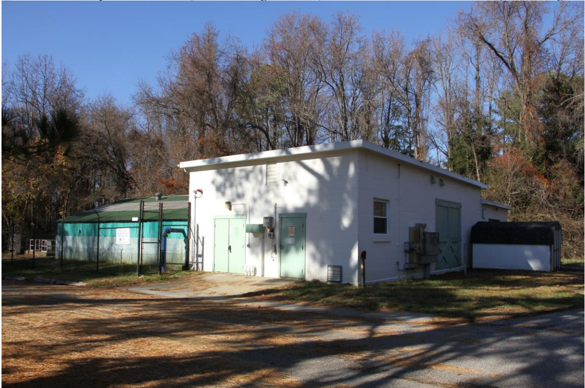
Photo 18 of 39: East College Parkway Area, Water Treatment Plant and Shed, south and east elevations, looking northwest
