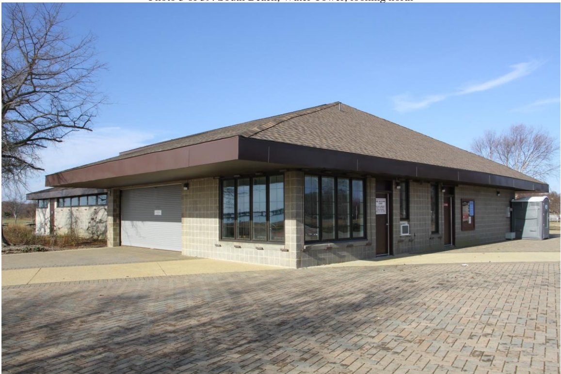
Photo 4 of 39: South Beach, Bathhouse and First Aid Station, south elevation and east façade, looking northwest
